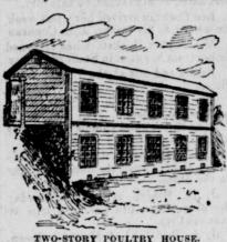
soil should be either naturally or artificially well drained, and the wall around the ends and back side of the lower story should be well made, so as to keep the interior from becoming damp. This wall can be built of rough stone, perhaps, more cheaply than of any other suitable material, where stones are plentiful.
