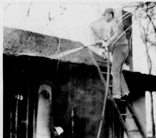
SMOKE SCREEN--Through the smoke screen, firemen drench the roof of the Raymond Precure home which was heavily damaged by fire Friday afternoon.
