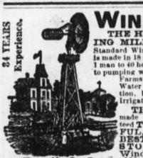
THE HALLADAY PUMP-ING MILL is acknowledged the Standard Wind Mill of the World and is made in 18 sizes, 8 to 60 ft. diameter, I man to 40 horse power. It is adapted to pumping water for Stock and Dairy Water for Stock and Dairy Farms, Ornamental and Village Water Supply and Fire Protec-tion, Railway Water Stations, Irrigation, Drainage, etc.
