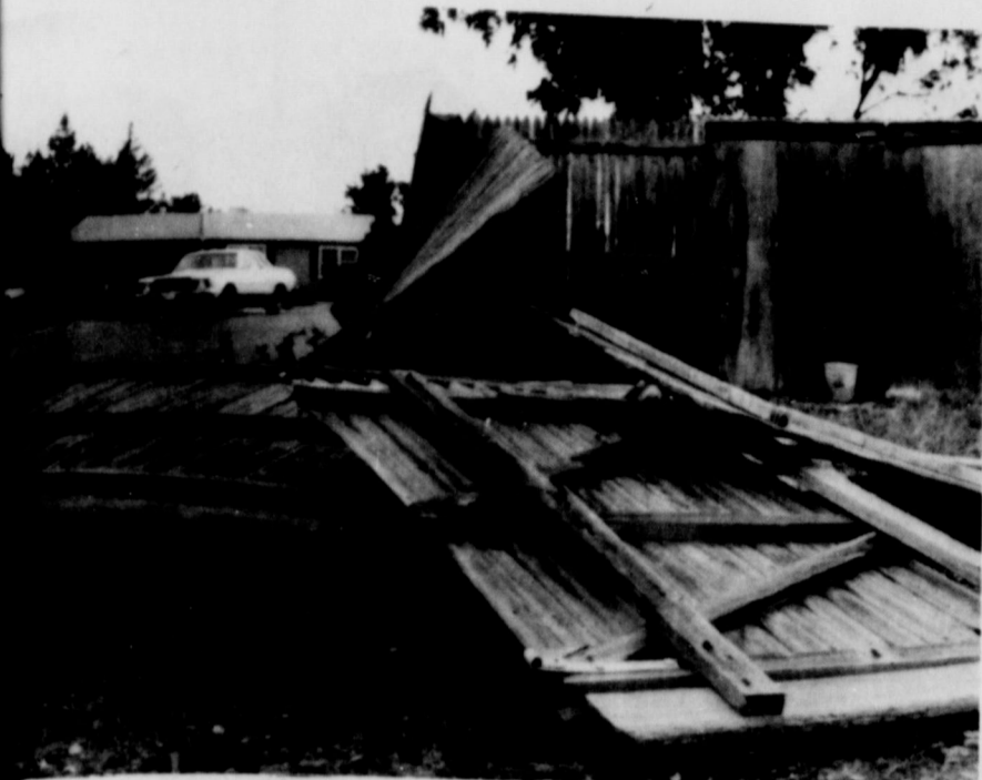
DAMAGE -- This section of fence at the Barry Weaver home, 4th and Ave. R, was typical of fencing in Tahoka after last Saturday night's high winds caused widespread damage.
