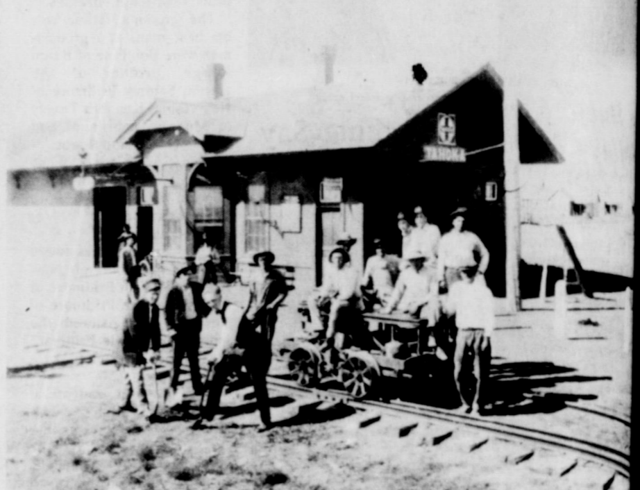
THE TOWN HISTORIANS say the Santa Fe Depot was built in 1910, and that marked the beginning of the building in Tahoka, especially the brick structures, because the bricks had to be shipped in. In the above picture, from left to right, are: Joe Heare, agent; Ivan Ewing, messenger; and Homer St. Clair, clerk. Tom Higgins is near center window. (Picture loaned by Frank Hill)
