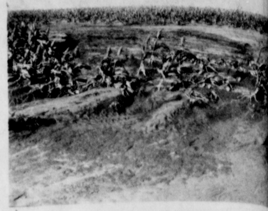
A SYSTEM OF PARALLEL TERRACES will catch and nearly all of the 18-inch average yearly rainfall in Lynn County. This is equal to 78,000,000 gallons of water per quarter section. An irrigation well would have to pump 1 GPM for 181 days to equal the average rainfall. Most Lynn County have irrigation only or have neither terraces or irrigation. Does your 78,000,000 gallons of water run down the bar ditch each year? See your Soil Conservation office in Tahoka. We can help.
