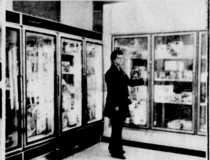
RIM ROCK'S NEW BUILDING features a 9x11 display freezer and two coolers, 10x26 and 12x12.
