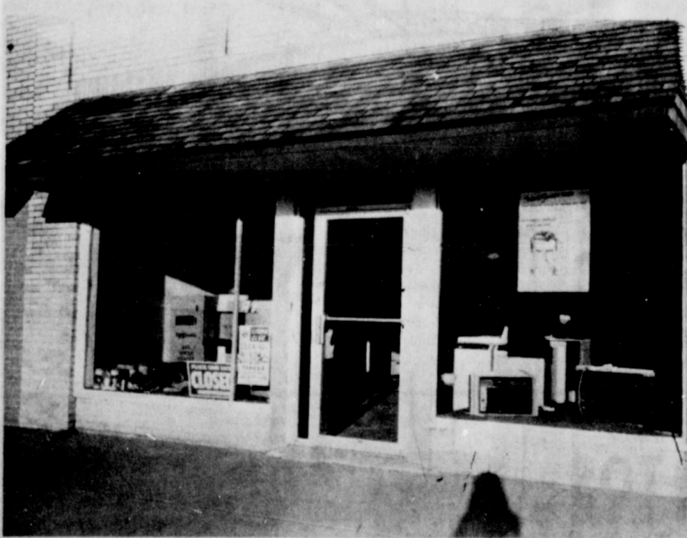
PROPRIETORS OF STICE REFRIGERATION in Tahoka have just completed a new face-lift job for their building.
