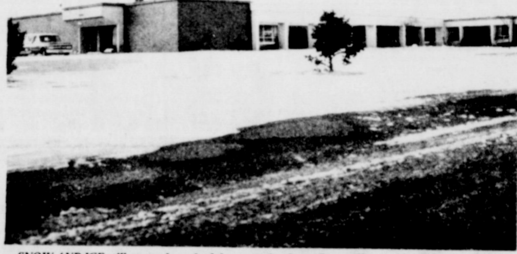
SNOW AND ICE still covered much of the ground at Lynn County Hospital late Monday. Low temperatures on Monday night and early Tuesday kept hazardous conditions on sidewalks and streets.
