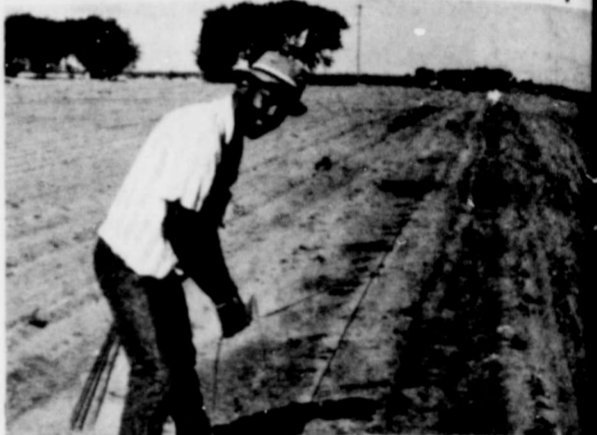
SETTING UP STAKES - Pictured above is Johnny Martin, summer aid with the Soil Conservation Service, setting stakes to prepare grid map.
