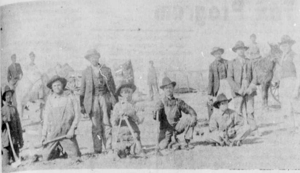
GRUBBING CREW is pictured above, probably working on road bed for railroad which was built here in 1910. (Floyce Sherrod photo)
