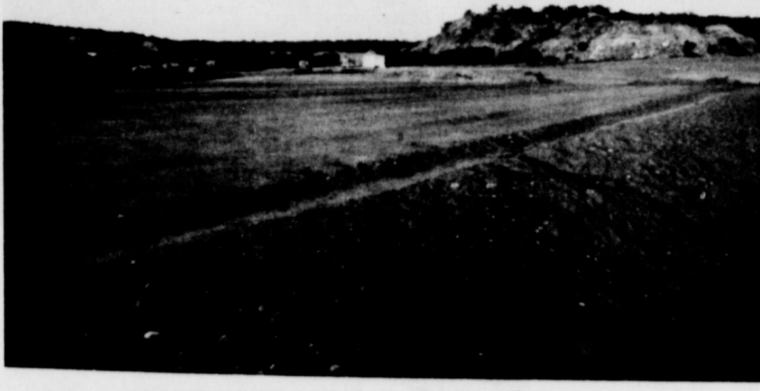
WORK AT COPPER BREAKS STATE PARK —This picture taken Sunday afternoon was made from atop the dam which is being built on Devis Creek in Copper Breaks State Park north of Crowell. The office and equipment of the contractor is visible in the background.
