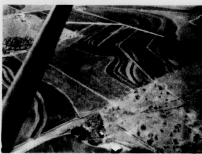
The above photo shows new parallel terraces emptying into a well-established waterway. Note the old conventional terraces have been removed, so there will be no interference with the new system. (SCS photo.)
