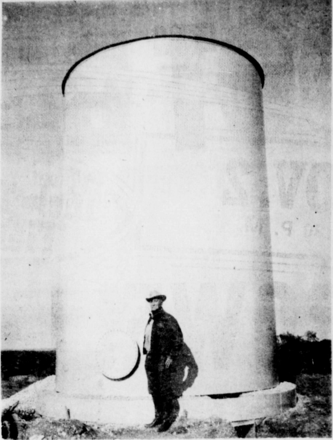
18,000-GALLON STORAGE TANK —George Self is pictured above standing by an 18,000-gallon storage tank located atop a hill on the Self property west of Crowell. Water stored in this tank will flow by gravity to areas west and south.
