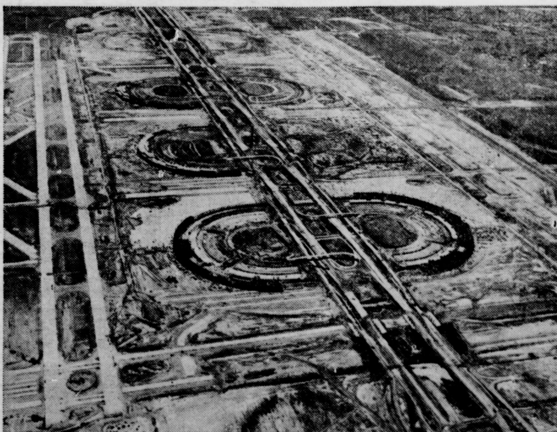
TEXAS-SIZE SUPERPORT —This aerial view of the new Dallas/Fort Worth Airport shows construction progress on the giant superport scheduled for opening in early fall, 1973. Conveniently located 17 miles from both Dallas and Fort Worth, the new airport is designed with the passenger in mind. Drive to gate boarding, close-in parking and simplified terminal procedures are only a few of the ultra modern features designed into the unique facility.
