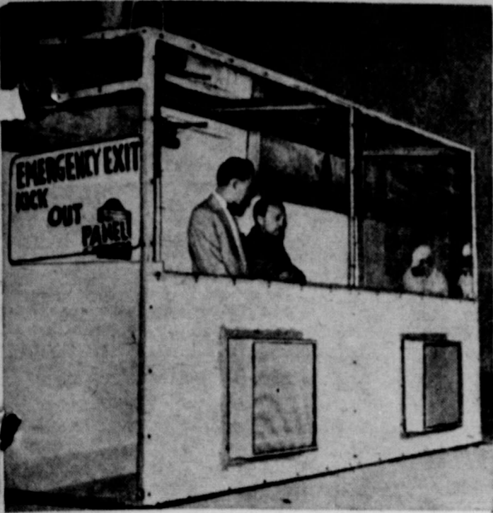
RADIOACTIVE ANSWER BOOTH —Its viewing windows constructed of 1/4-inch-thick glasslike plastic, this atomic isolation booth permits persons to observe separation of plutonium from uranium fuel substances at the Hanford Atomic Plant, Richland, Wash. Shadows of conventionally garbed workers can be seen reflected in window at far right. Air for observers is pumped in from outside the windowless concrete building in which booth is located.
