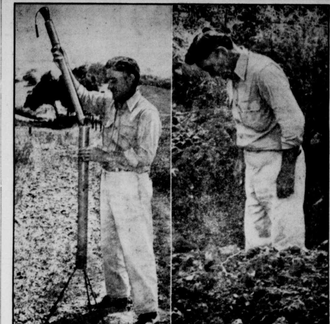
FOXHOLE IN 90 SECONDS—G.I.'s should welcome this new device—a "90-Second Foxhole Digger," developed by the Stanford Research Institute of Menlo Park, Calif. The Digger enables ground troops to dig their positions in a minimum warning period. Left, a technician places the rocket-explosive unit in a launching tube. After the fuse is ignited, the technician takes cover, and the rocket is driven about two feet into the ground. The charges explode and—presto—a four-foot deep, four-foot wide crater is cleared, right.
