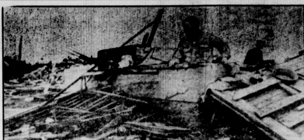
SEA OF DESTRUCTION—Captain Virgil Bailey, 34, of Falkville, Ala., stands at the prow of the good ship Storm Cellar, surveys the sea of destruction which poured over him while he was safely below decks. At least three persons were killed and many buildings leveled along the storm's path.
