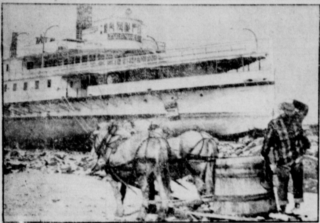
HAZARD TO NAVIGATION —A "sap" at the helm has imperiled many a ship, but this is perhaps the first time that tree sap has proved a hazard to a steamship's progress. The 49-year-old Ticonderoga, making a 9000-foot overland journey from Lake Champlain to the Shelburne, Vt., Museum, is encountered by Farmer Denny Waller, who is making the rounds of his sugar bush with his sap-collection rig. Maple sap running free means "spring thaw," and spring thaw means that the last of the Lake Champlain sidewheelers may hang up on a mud bank before she can complete the journey to her final berth on the museum's grounds.
