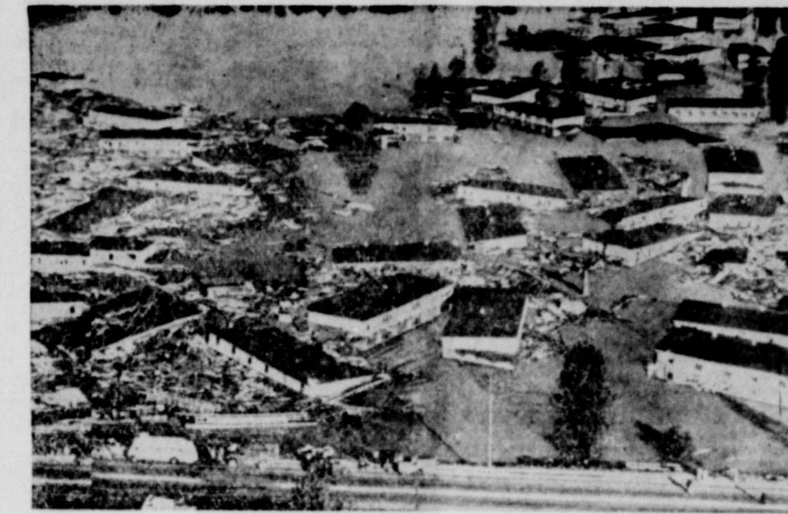
COLUMBIA RIVER DESTROYS OREGON CITY... This aerial view shows what is left of the war-built city of Vaport, Ore., after a dyke of the swollen Columbia river broke and let the flood waters pour destructively through. Homes were ripped from their foundations and smashed against one wall of the town as the flood ripped through the community, leaving 19,000 Vaport residents homeless and many others drowned. Elsewhere, vast areas of Oregon and Washington also were flooded by the rampaging Columbia. An approximate 90,000 persons were made homeless throughout the Pacific Northwest and the damage toll was at least 75 billion dollars.
