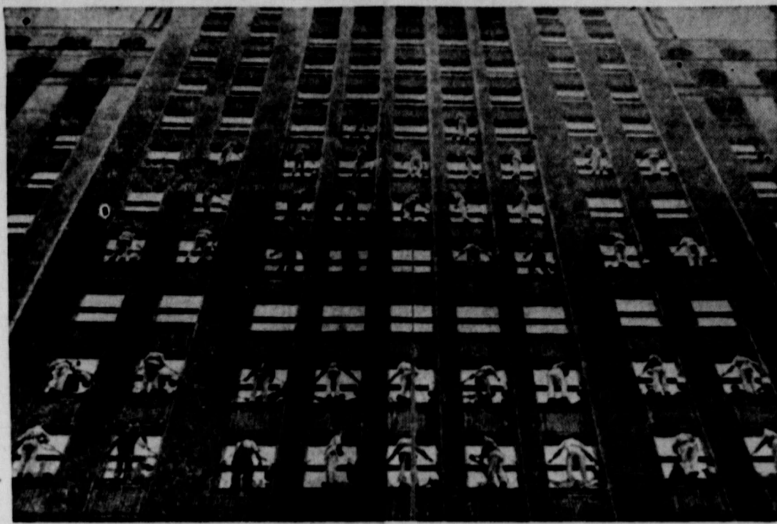
NO SECOND-STORY MEN, THEY... This modern age of steel-thewed skyscrapers with thousands of windows is the cause of situations like the one recorded here. It was touted as the largest mass window-washing job ever to be held, and it took place on the impressive face of the world's largest commercial building, the Merchandise Mart in Chicago. The event, which made even hardened city dwellers look up for a few moments, took place during a clean up campaign in Chicago. Between 300 and 400 window washers, provided by their association from all parts of the city, took part in the demonstration.
