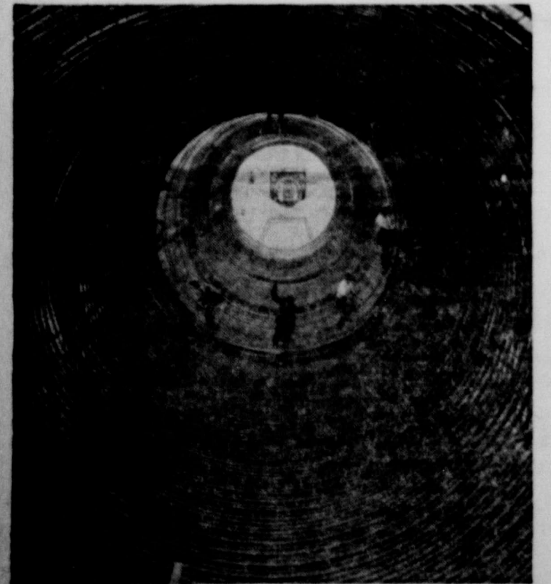
COLUMBIA BASIN SIPHON ... Near Adrian, Wash., steel workers were set of heavy reinforcing bars around which will be poured concrete for Crab creek inverted siphons which will convey Columbia basin irrigation water across Dry Gulch to reclaim eastern Washington overbrush land. Twenty-five feet in diameter and 8,100 feet long, it will be world's largest monolithic concrete siphon.
