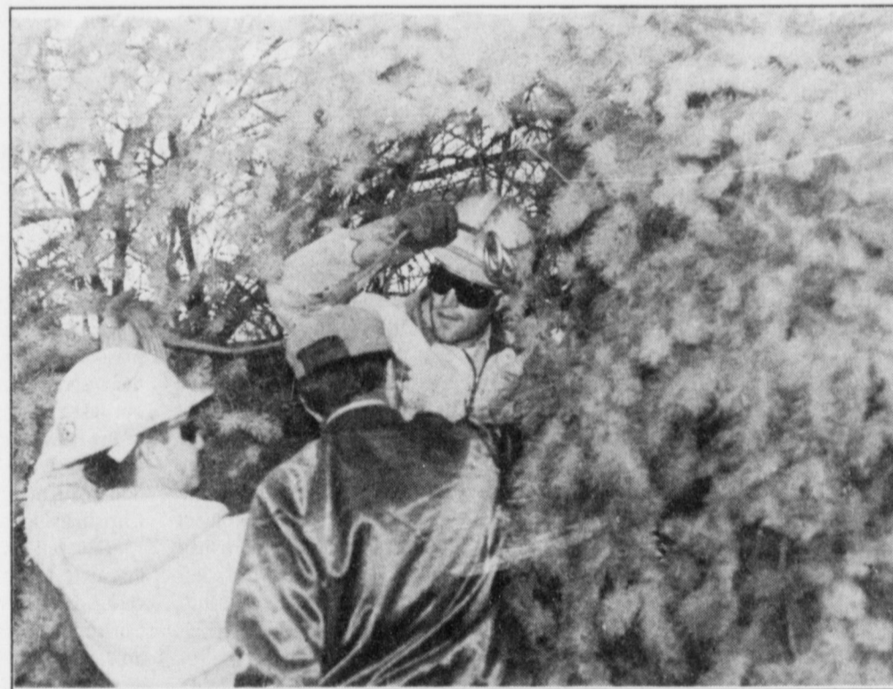
Bailey County Electric workers Scott Miramontes (left) and Kip McCall attach a cable to a giant Christmas tree. Several local companies helped put up the 40-foot spruce in the Mule lot Wednesday morning.
