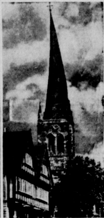
CROOKED SPIRE . . . The famous crooked spire of the parish church, Chesterfield, England. The spire is twisted owing to the warping of the timbers beneath a leaden covering. It is 230 feet high, 8 feet out of perpendicular.
