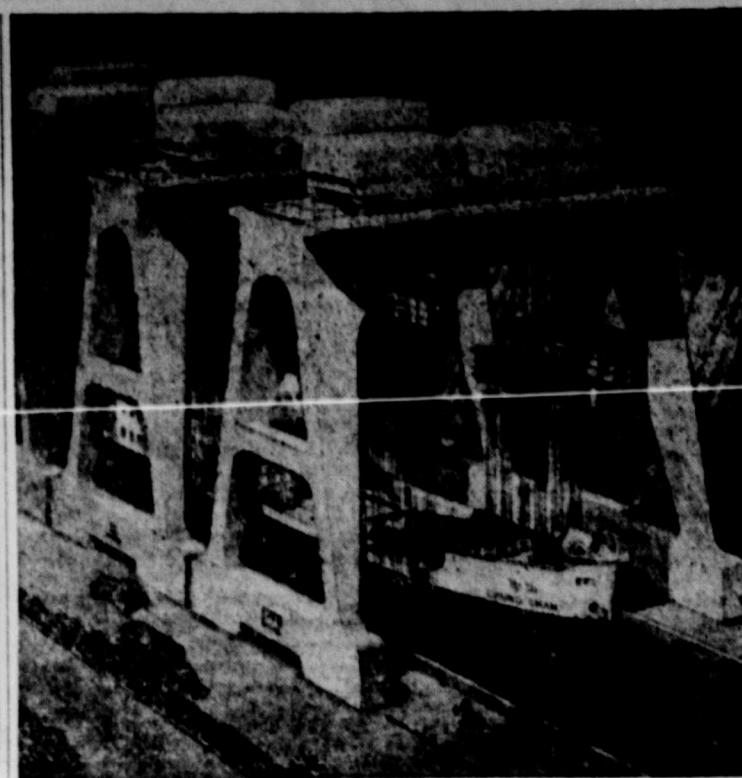
MORE POWER TO THE DRAGON . . . China is to pump new life into the old dragon by building the biggest concrete dam, irrigation project and power plant ever known. Yangtze gorge project, with co-operation of the U. S. bureau of reclamation, builder of Boulder and Grand Coulee dams, is drafting overall plans. The mechanical lock facilities are shown above. They are capable of holding a loaded vessel of several thousand tons displacement capacity. John Lucian Savage is consulting engineer.
