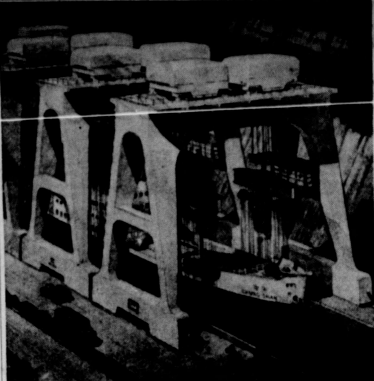
MORE POWER TO THE DRAGON . . . China is to pump new life into the old dragon by building the biggest concrete dam, irrigation project and power plant ever known. Yangtze gorge project, with co-operation of the U. S. bureau of reclamation, builder of Boulder and Grand Coulee dams, is drafting overall plans. The mechanical lock facilities are shown above. They are capable of hoisting a loaded vessel of several thousand tons displacement capacity. John Lucian Savage is consulting engineer.
