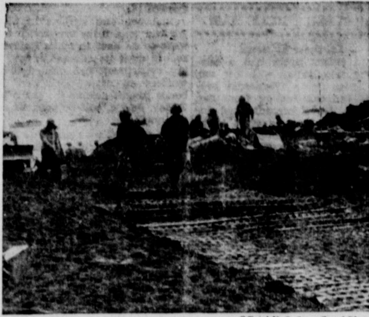
Official U. S. Coast Guard Photo Bulldozer prepares to widen a roadway from the terra-cotta Jima beach. The steel matting provides a firm road-bed, over the soft volcanic ash, to a supply dump further inland. This is one of the many handicaps being overcome by our soldiers and made possible through equipment purchased by War Bonds. Start saving now for the Mighty 7th War Loan opening May 14. From U. S. Treasury
