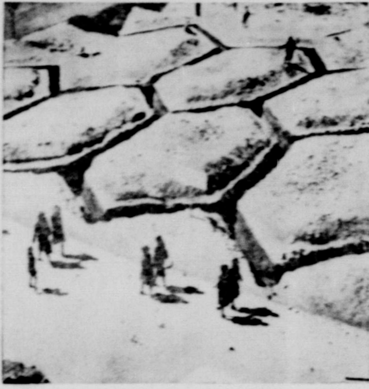
The still trenches that cut up an area "some place in Italy" in a waffle-like pattern are being used by the Air WAC's stationed near the headquarters of the 13th Air Force in Italy. This new type of trench is said to offer considerably more protection, and is harder to hit from air.
