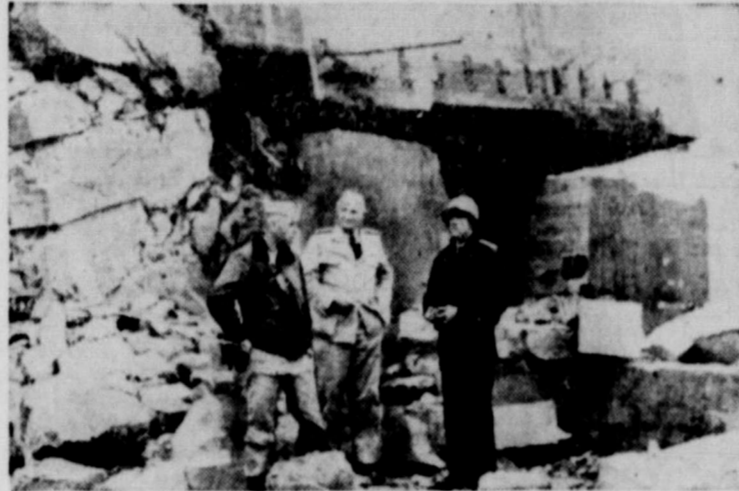
Three American naval officers stand amid the wreckage of the arsenal at Cherbourg, graphic testimony to the efficiency of German demolition squads. Left to right are Commodore William A. Sullivan, port salvage expert; Rear Adm. John Wilkes; and Rear Adm. Alan Kirk, commander of U. S. naval task forces in French waters.
