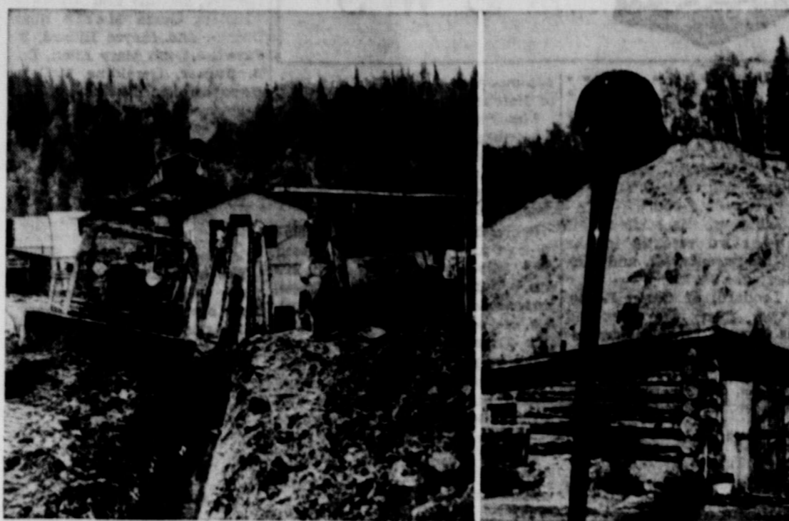
Ten thousand square miles of prehistoric, mineral-rich oil sands in Alberta, Canada, will provide the United Nations with huge quantities of oil. Experimental production has been in effect for more than a year at McMurray, 300 miles northeast of Edmonton. Photos show (left) conveyor belts carrying oil sands to the separation plant where, through flotation, hot water washes oil free from sand. Right: "Black gold" flows freely through the pipeline after the separation process is completed.
