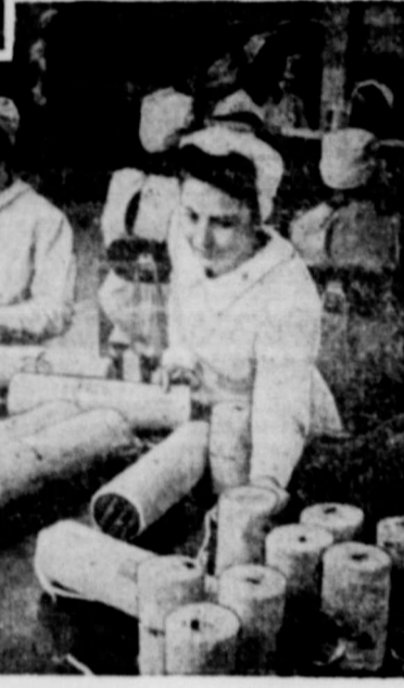
No, these men are not bakers pouring butter into pie—It's TNT, one of the deadliest explosives known, being poured into shells.
