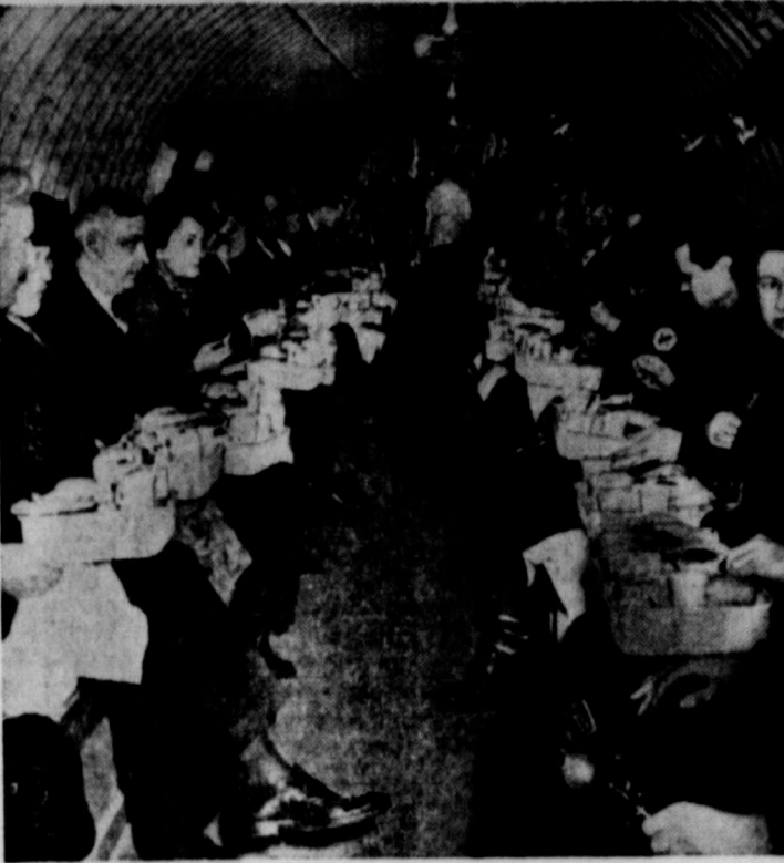
A luncheon served on air line trays publicly opened the bomb shelter by a large rubber concern at Akron, Ohio. This is a shatterproof flexible structure of the type tested by the war department. It is made of strong congealed plates forming a gas and water-tight cylinder, and is large enough to accommodate 50 people.
