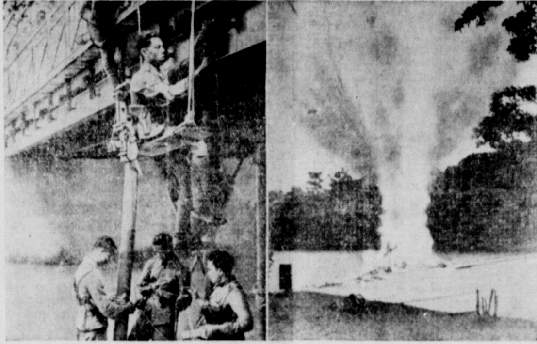
In the United States an ordinary railroad line would count its bridges and trestles by the scores or by the hundreds. In Java they are numbered in the thousands. Bridges are seen everywhere spanning rivers and ravines. And so, before Java fell to the invading Japs, the Netherlands East Indies mountain army became expert in demolition. At left they are seen as they mined a bridge. Right: A small pontoon bridge for infantry crossing is shown as it was destroyed by a well-placed shell.
