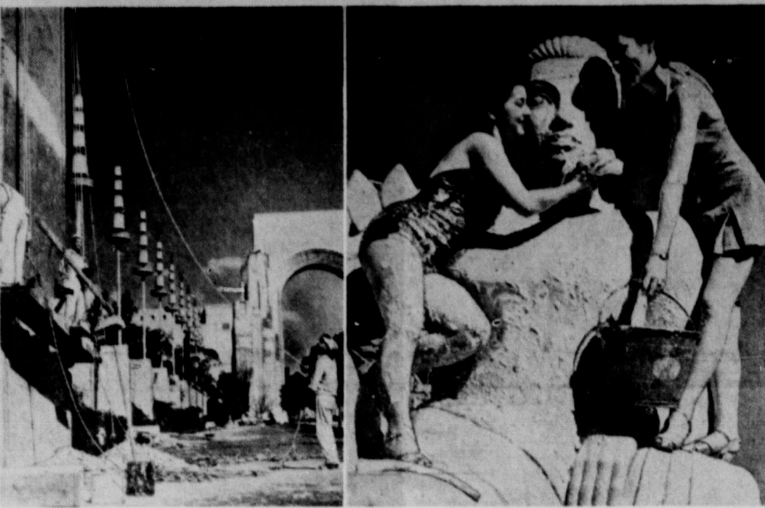
Face-lifting operations for the 1940 Golden Gate International exposition are well under way in preparation for the opening day, May 25. Left: Workmen are pictured plastering and painting in Treasure Island's court of reflections, where an entirely new color scheme will greet first-day visitors. Right: Statuary gets a bath on the exposition grounds. Jeanette Adams and Fay Lacey do their share with this sculptured figure.
