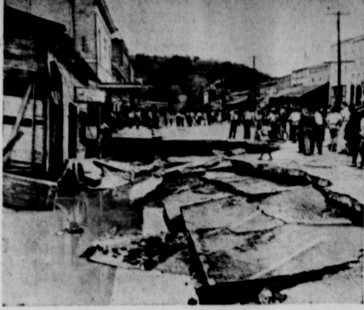
Undermined by flood waters from a swollen tributary of the Alabama river, this section of the Prattville, Ala., main street collapsed, halting traffic through the business district. Floods were caused by heavy rains, and though there was no loss of life, more than 3,000 persons in the southern part of the state were forced to flee their homes.
