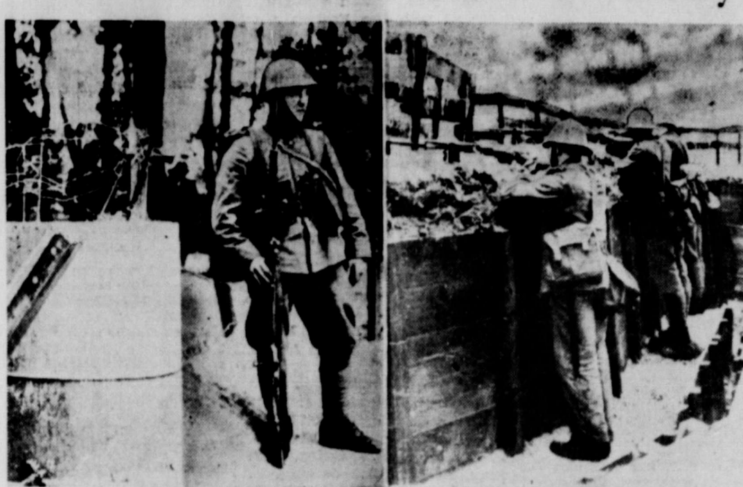
"Somewhere in Holland too close to Germany" is the only locality identification given for this show of Dutch preparedness on the German border. Left: A steel-helmeted sentry stands guard before the entrance to one of the new border fortresses. The concrete slab is a "tank stopper," garnished with steel rails and a bouquet of barbed wire. Right: Soldiers of the Netherlands' regular army stand guard in a trench along the German border. Such scenes are plentiful along the entire frontier.
