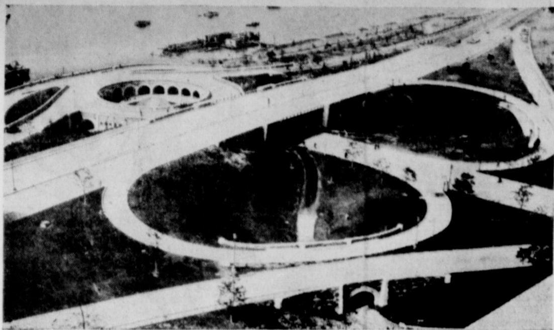
An elevation view of the traffic circle and fountain at Seventy-ninth street, New York city, showing part of the superhighway that is a big feature of the $24,000,000 improvement project on Manhattan's west side waterfront. Beneath this traffic circle is a garage accommodating 250 cars. A yacht basin and a promenade are other features yet to be completed.
