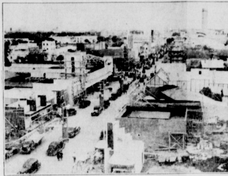
Called by showmen "the greatest Midway in World's Fair history," the $5,000,000 Texas Centennial is racing to completion and readiness for the June 6 opening day in Dallas.
