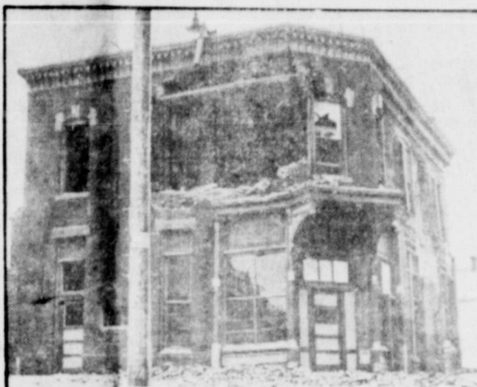
Undaunted by new earthquakes which swelled to more than 700 the number of tremors which have shaken the city since Oct. 12, taking several lives and immense toll of property, residents of Helena, Mont., have launched the task of rebuilding numerous wrecked structures, such as those shown above. When the smokestack crashed down on the brewery shown at top, two men were killed. In the pioneer building shown below, a quake ripped away almost half the side wall.
