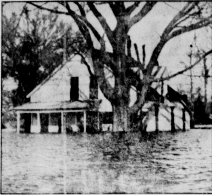
When flood waters of the Black and White rivers merged at Newport, Ark., a gray outlook resulted for the owner of this home. From a depth of six feet when this photo was taken, the waters rose to 12 feet later in the day.
