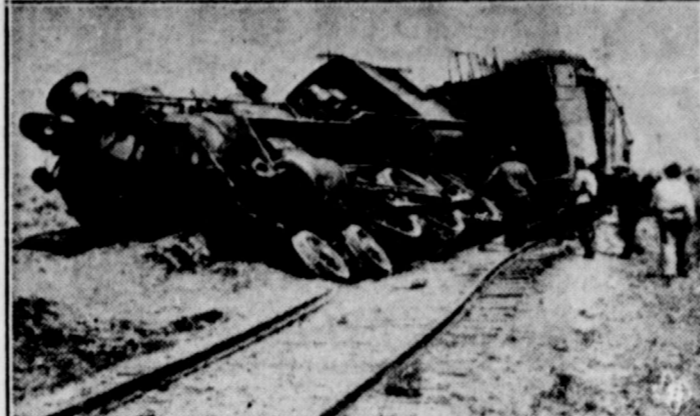
The photo above shows the wreck of the Quanah, Acme and Pacific train west of Paducah, Texas, caused by a four-inch rain that undermined the track. The engine quit the rails and rode cross-ties for 300 feet before it overturned, as shown in this splendid picture. The engineer and fireman stayed with the cab and were injured. Traffic was delayed 16 hours on the line. (Texas News Photos.)
