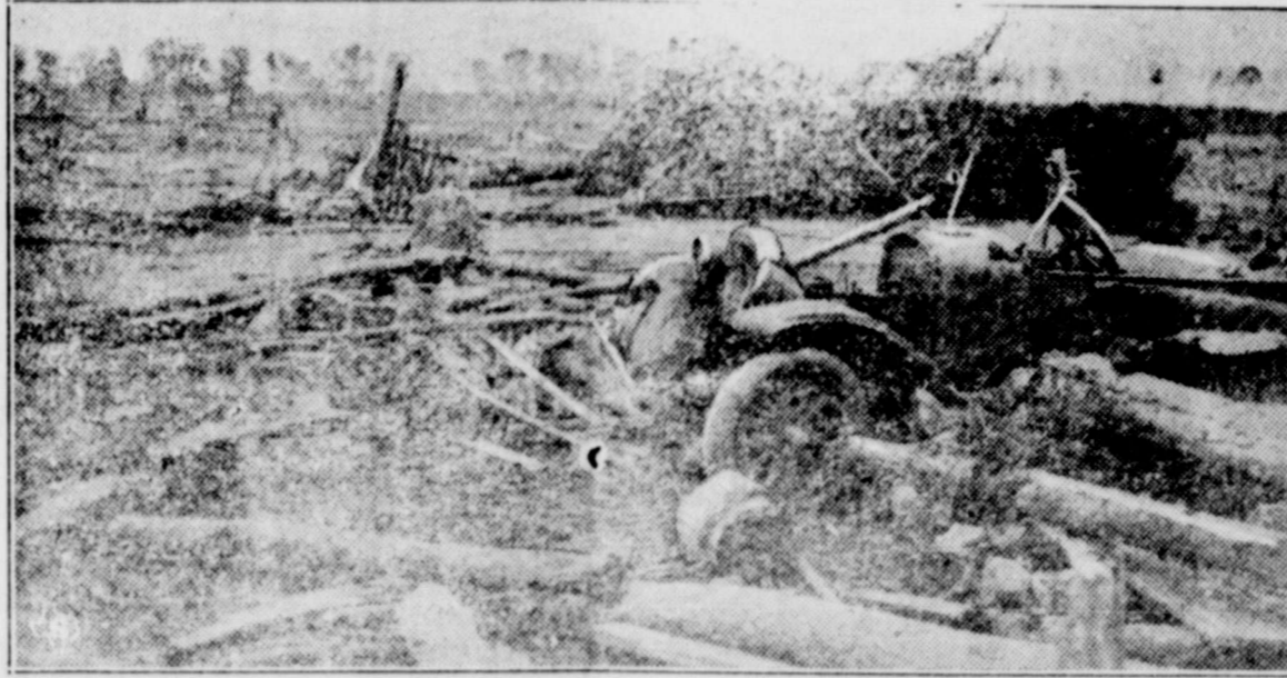
Two persons were killed instantly, and fifty more injured, several probably fatally when a new tornado struck East Texas, this time in the Bowie county plantation section. Above is one of the typical scenes in the cyclone's path. About 20 tenant houses were lifted from their foundations and scattered over the fields of young cotton. Livestock and crops were damaged.
