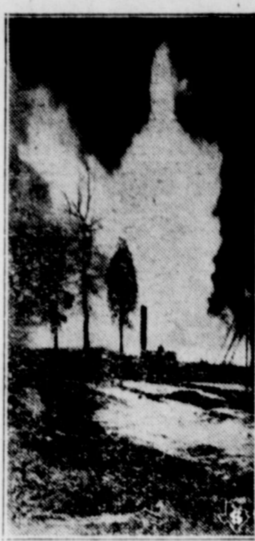
This great sheet of flame, roaring 200 feet in the air, is the Mad-dy No. 1 well in the Conroe field, north of Houston, which has been burning for nearly two weeks. A crater more than 200 feet wide has defied all efforts to check the wild flames.
