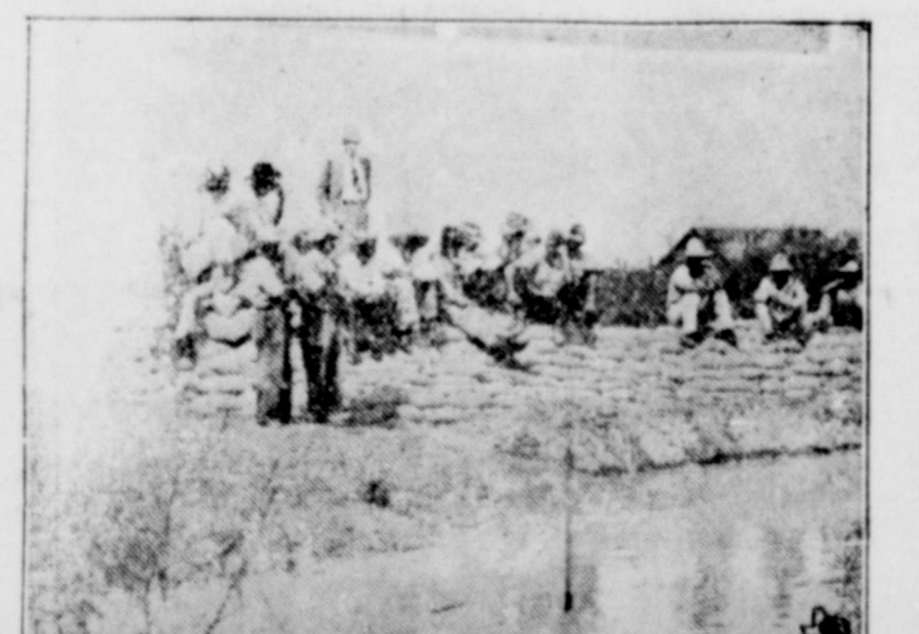
Scenes like this were common in the Lower Rio Grande valley when the Rio Grande flooded thousands of acres of rich citrus land. Here is the hurriedly constructed sand bag levee in a railroad cut south of McAllen, Texas, with Mexican laborers watching, that they might stop any leak which might appear.
