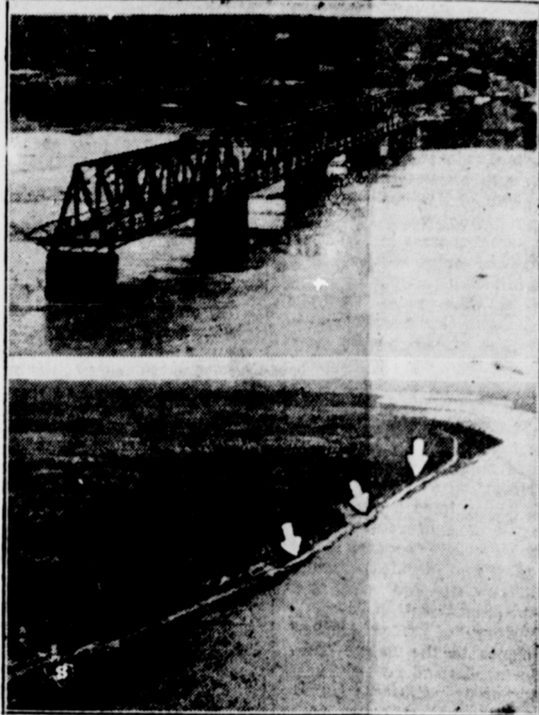
The top photo is a closeup aerial photo of the bridge over the Rio Grande river showing how the middle spans were washed away by debris piling up against them as the muddy waters swept toward the sea. Below is a section of the Southern Pacific tracks near Del Rio, inundated by the Rio Grande.
