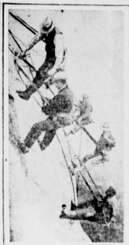
On the rocky face of Mount Rushmore, in western South Dakota, workmen with air-hammers are sculpturing the faces of four presidents as part of a gigantic memorial designed by Gutzon Borglum. The photograph at left shows vividly the difficulties of the task. Borglum is shown at right opposite a model of the group.
