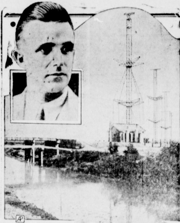
The pagoda-like construction of the antenna towers of the new Chinese radio station at Shanghai was added to give strength to the steel masts. George F. Shekelen (inset), San Francisco, is assisting in the operation of the station.
