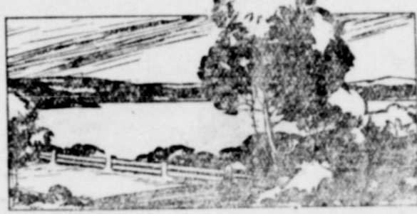
A view of the 20,000,000-gallon lake that was built to cool the compressor engines at Brad.
