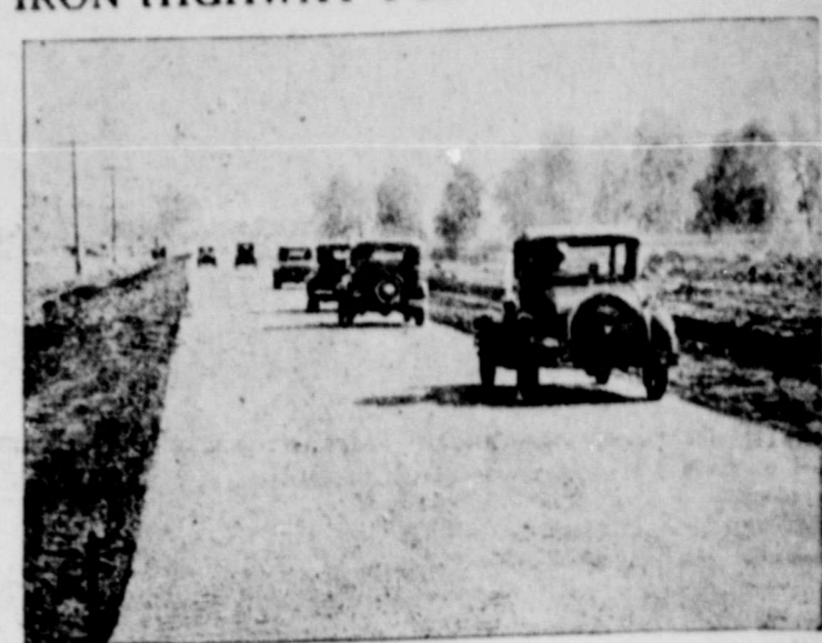
This is an experimental section of iron highway in Sangamon county, near Springfield, Ill. Bricks are laid on metal sheets.
