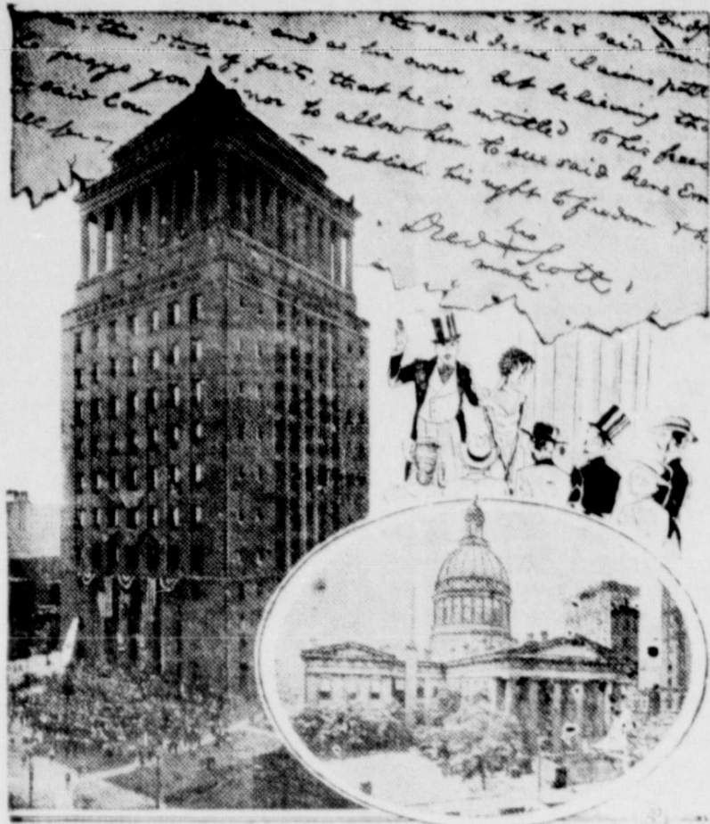
St. Louis' historic courthouse (lower right) has been abandoned for a new $4,500,000 structure (left). Slaves once were auctioned on the steps of the old building and the famous Dred Scott case heard there, where Scott's mark (top right) is still on record.
