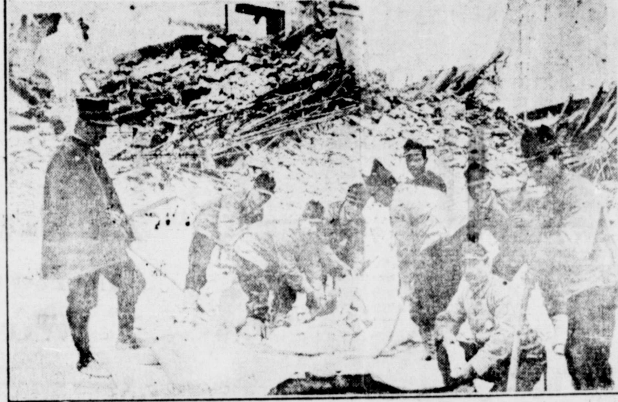
Thousands were killed when earthquakes destroyed towns in southern Italy. The disaster caused the most widespread death and devastation since the Messina earthquake of 1908 when 75,000 persons were killed. The pictures above were made following the Messina disaster. Upper picture shows buildings reduced to rubble. Below soldiers removing body of victim from wreckage.
