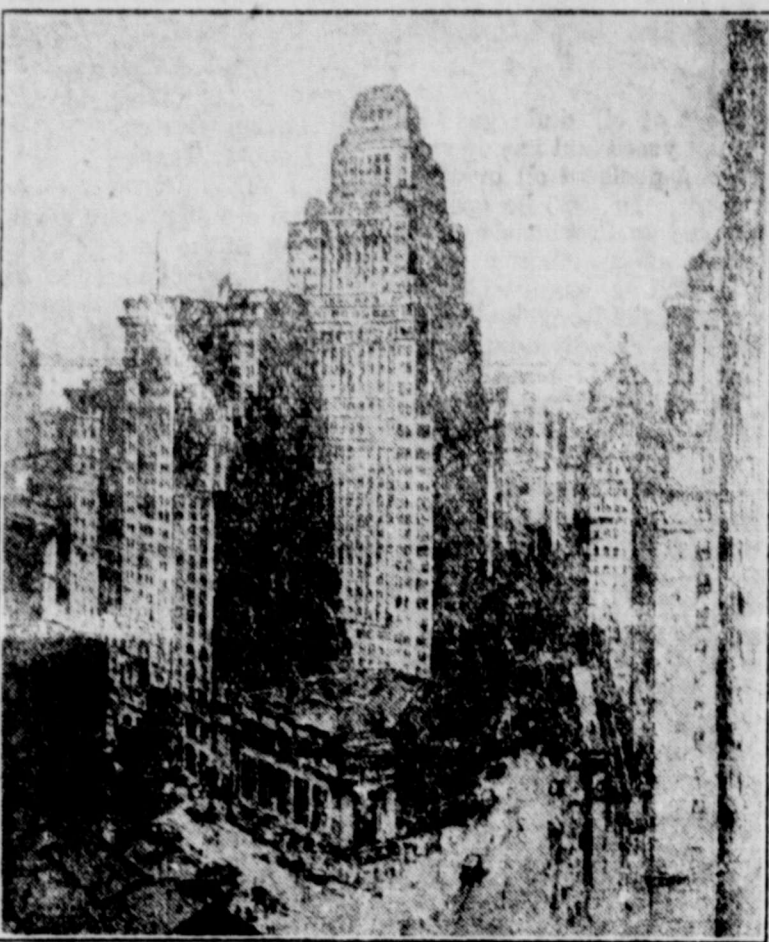
Anton Schütz' etching of new Equitable Trust Company Building, first American skyscraper to utilize new glass for admitting sun's vital rays indoors.
