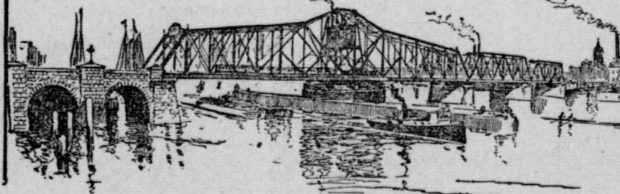
SIDE VIEW OF THE NEW FOUR-TRACK STEEL DRAW-BRIDGE OVER THE HARLEM RIVER.
