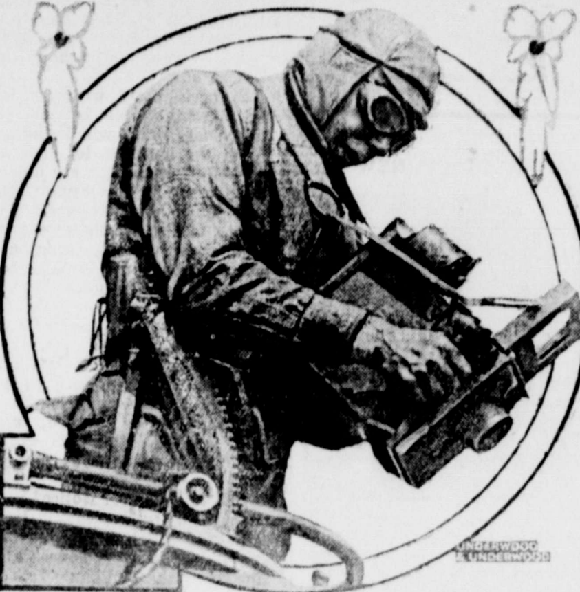
Frank Morris is here seen operating a movie camera from an airplane with his invention—the addition of a small motor driven by an 8-volt, 60-ampere battery which does away with the three cranks that the movie operator has to use and makes serial movie photography steady and easy.
